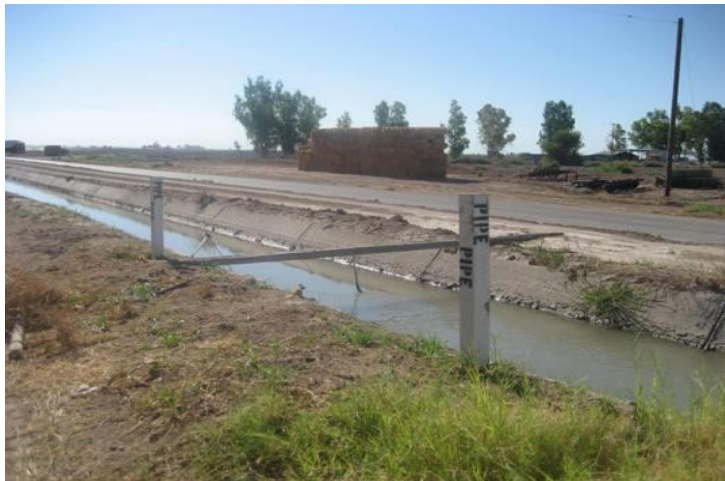
A marker indicating the location of a “Pipe” that leads to a residence. Typically, a “Pipe” stems from IID managed canal that leads to a cistern and a residential water pump which pressurizes the residence’s water supply. This is commonly referred to as the “Intake system.”
