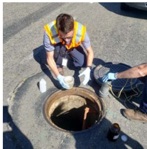
A wastewater authority employee collecting a water sample from our sewer
