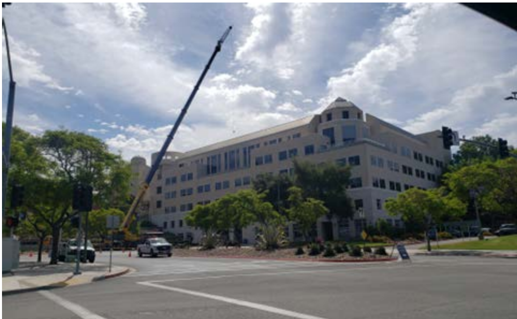
New Equipment being craned to the Elevator Machine Room
