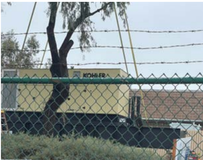
New Generator being set by a crane
