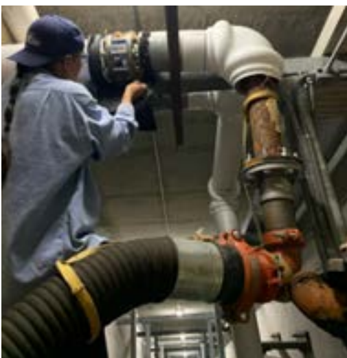
A Building Service Engineer diverting water to a storage container
