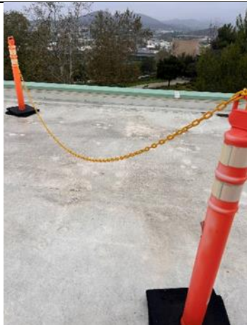
Photos taken by Safety, Health, and Sustainability October 17, 2025 and October 27, 2025
