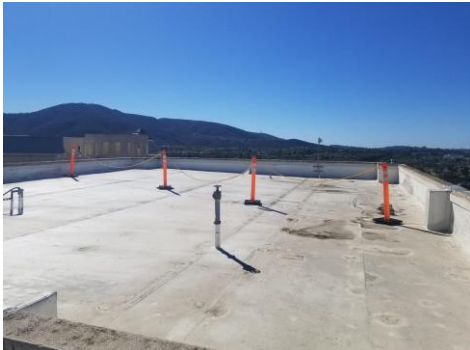
Image 2: Southwest Corner of building
