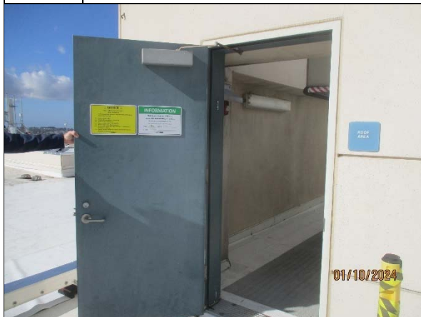
3. Rooftop Access Door (Locked)
