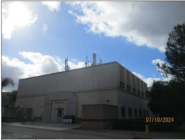
49. Verizon Sector D Ground View
