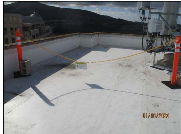
28. Verizon Sector B 13' Barrier w/ Caution Sign
