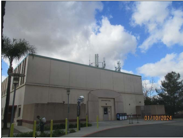
19. Verizon Sector A Ground View
