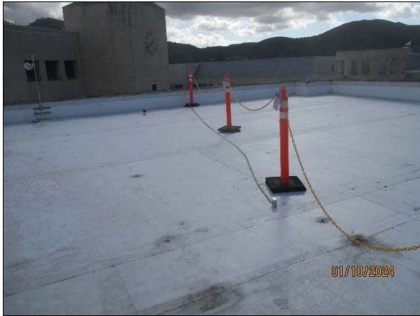
31. Verizon Sector B 38' Barrier w/ Notice Signs
