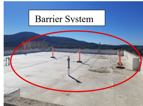
Image 2: Southwest Corner of building
