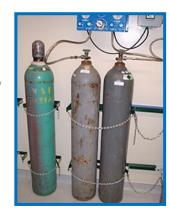
Nylon straps <u>may not</u> be used in place of chain restraints. C-clamp restraint systems are not allowed.
