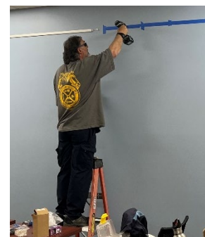
Patrick Pelonero, facilities maintenance mechanic, installs the framing system.
